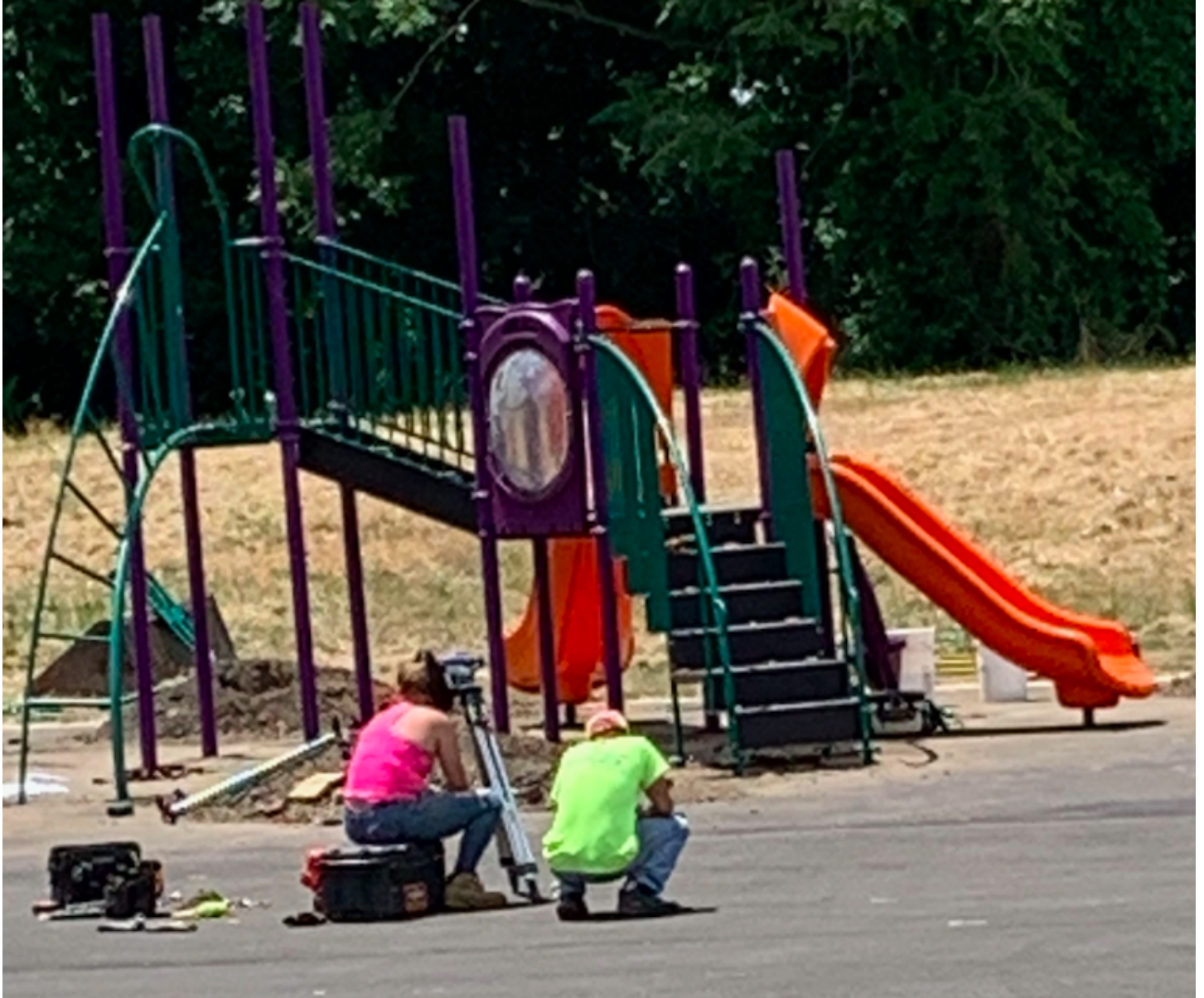
Playground Installation at E. W. Rhodes School
